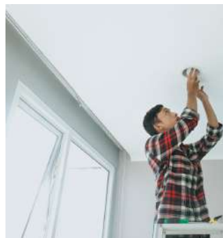
Gypsum/Fals e Ceiling Worker
